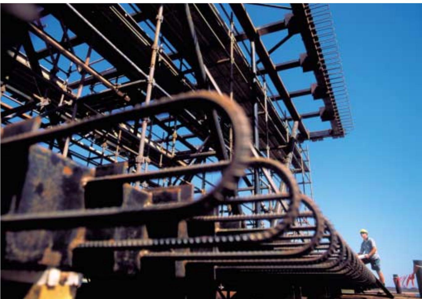
*Shell of the first fabricated steel cell to be used in construction of the wharf.*
